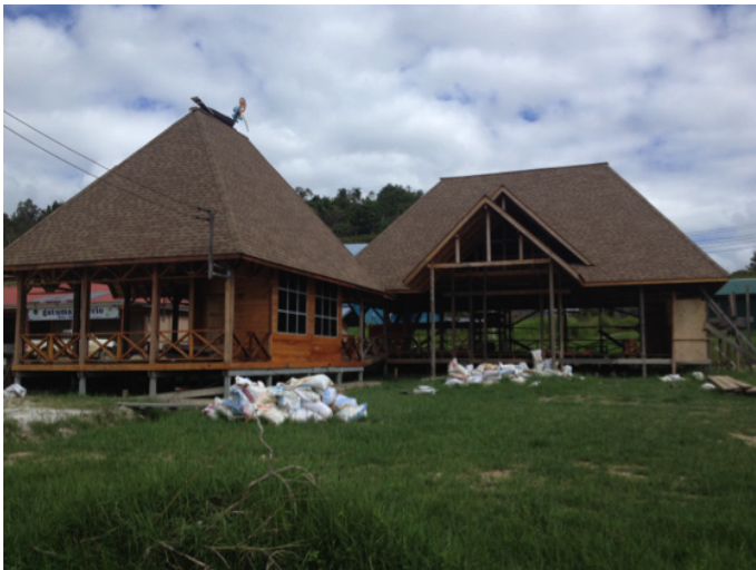
Image 1: Kelabit Highlands Community Museum building under construction, Bario, December 2015 (Kelly, 2015)
